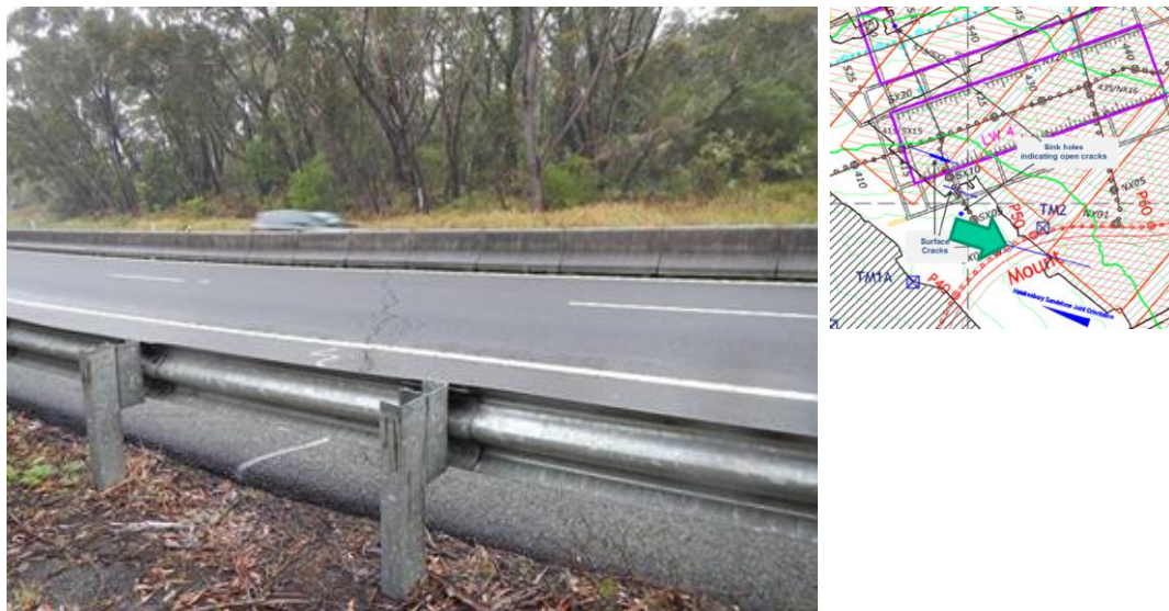
Figure 6: Cracks in the Pavement
