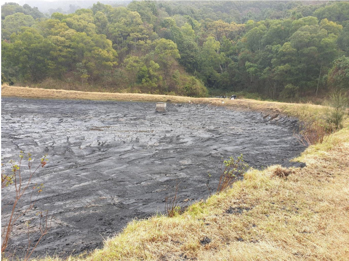
Figure 5 – Recently desilted dam near emplacement area
