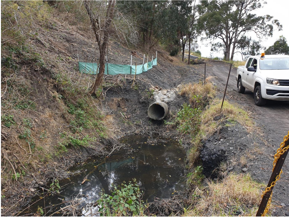
Plate 1 – Drain maintenance on access road within site
