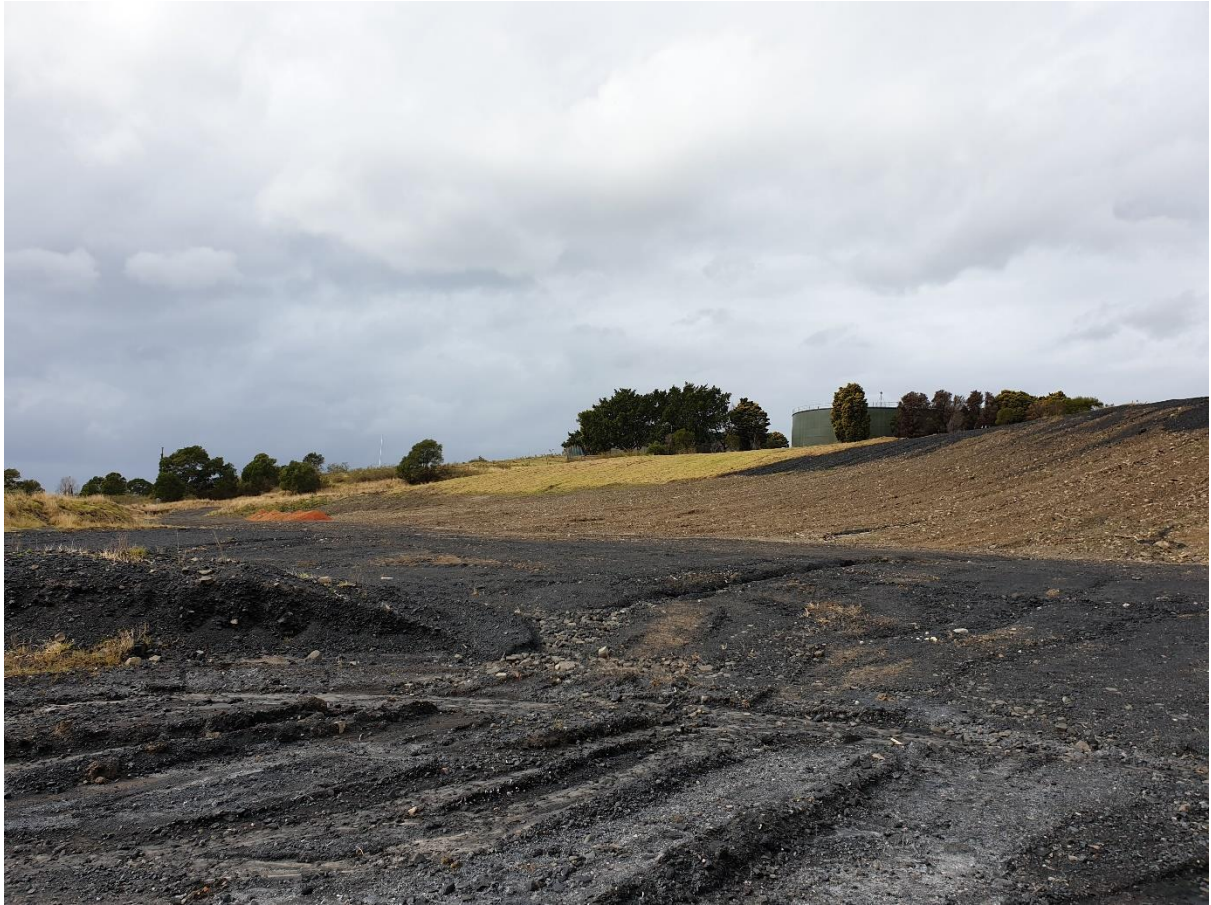
Plate 4 – Progressive rehabilitation including mulch and turf placement within the RVC site
