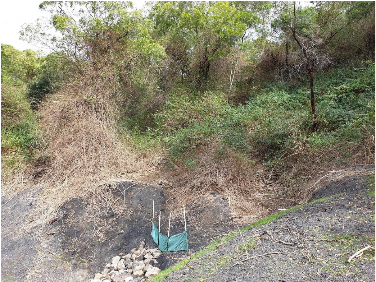
Plate 3 – Erosion and sediment control and weed removal within the site
